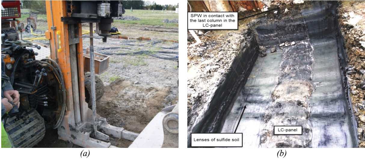
Fig. 3-7: (a) KPS test in LCC panel; (b) Excavated LCC panel 2.5 m below ground surface
